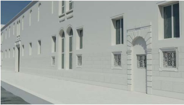
Figure 3: Details on the facade.
